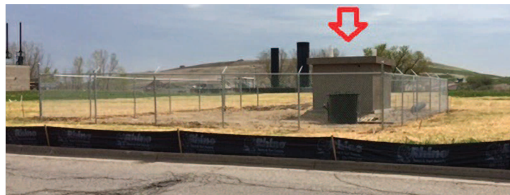
New sewer pumping station on east side of Giddings Rd. north of Silverbell Rd.
