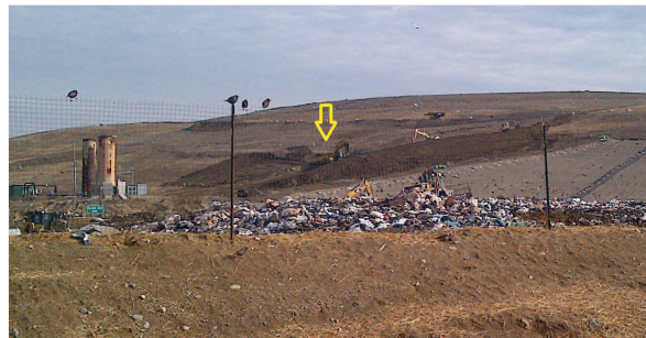
Excavation to remove sump pump from area west of old Cell 1
